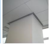
(2) Lockable & de-mountable double hook typhoon proof exterior ceiling in 4mm aluminium
